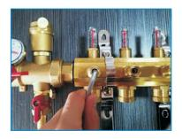
Automatic temperature control for every room is possible by installing electrical actuator normally closed or normally open. To install the electrical actuator you have to remove the handwheel of the shut-off valve
