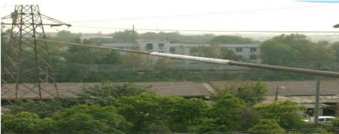
Intended use: To repair damaged conductor where up to all aluminum wires are broken.
