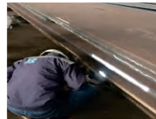
船检验原材料 Ship inspection of raw materials
