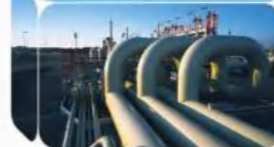
West-east gas pipeline
