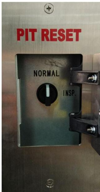
[Figure 7.3 PIT RESET DEVICE]
