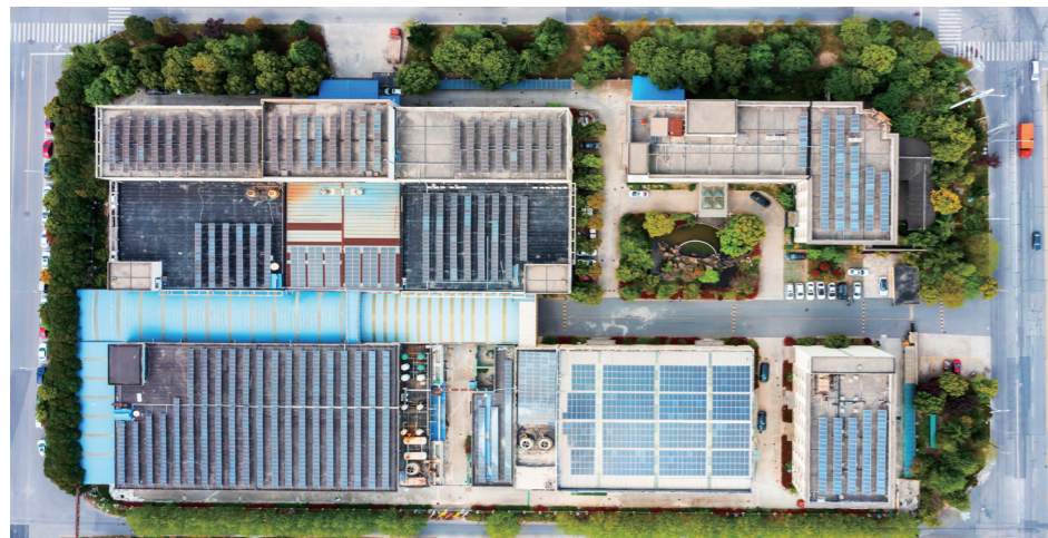
Whole-house solar power generation equipment, energy-saving and environmentally friendly for emission reduction.
