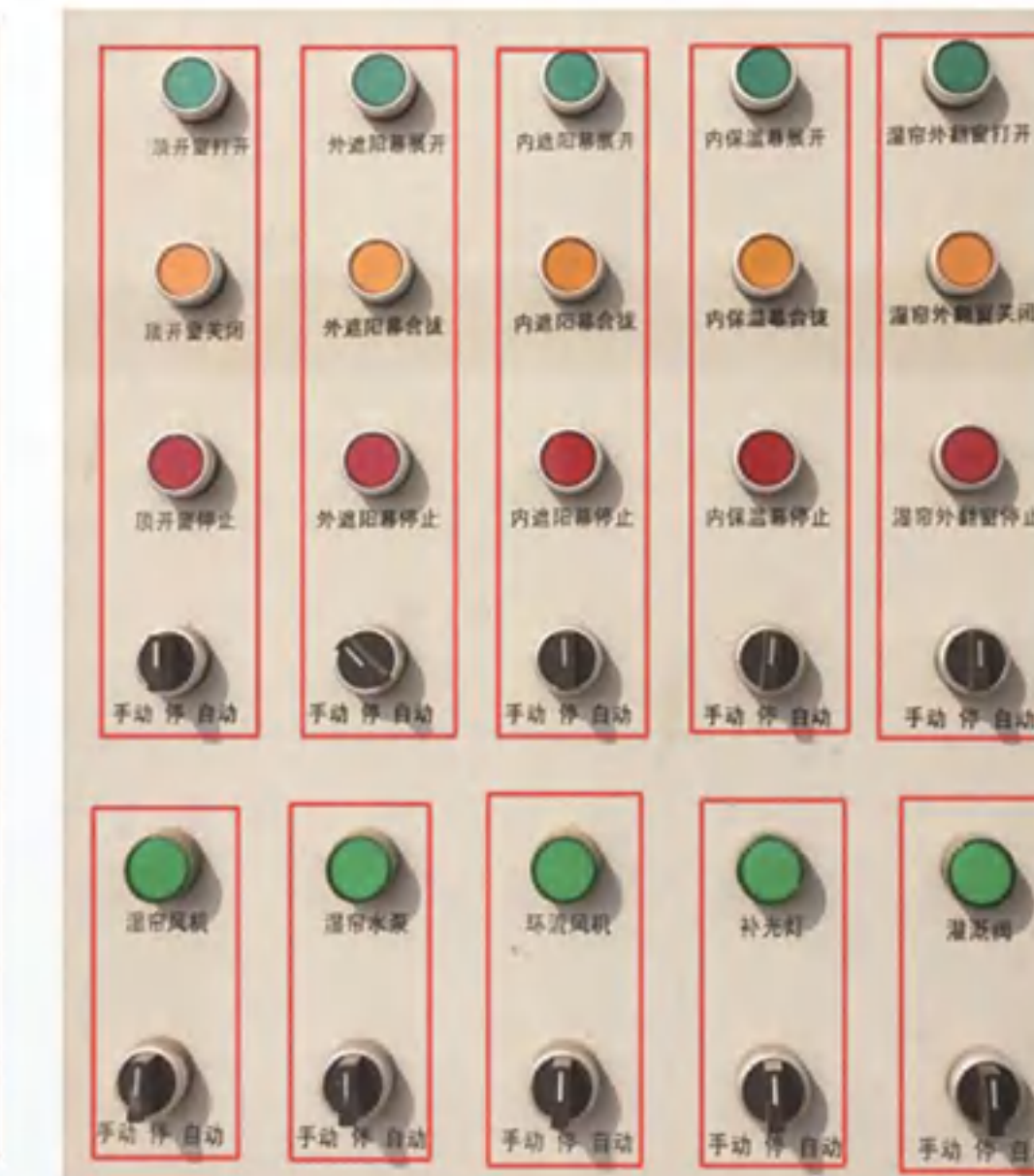
Wenluo type greenhouse IoT standard control cabinet panel
