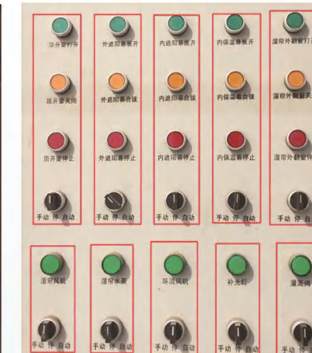
Wenluo type greenhouse IoT standard control cabinet panel
