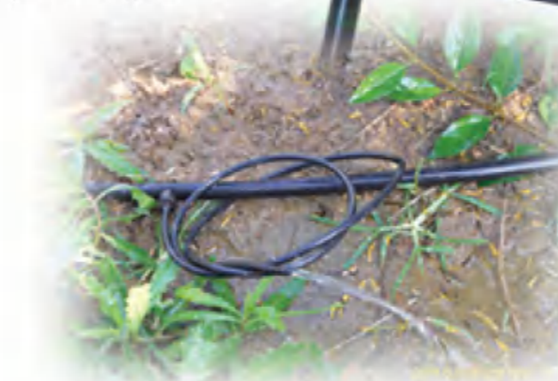
供水地下干管 main pipe underground
