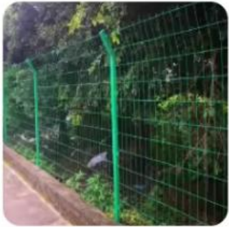
No barrier enclosure
