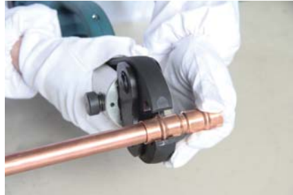
2.Insert the Press fittings into the end of the copper tube
