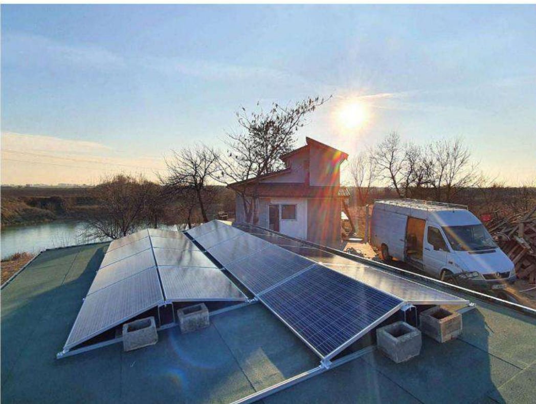
East & West Ballasted Mounting-Bulgaria
