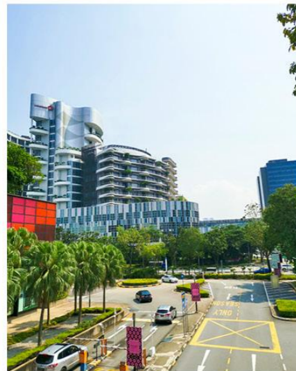
Singapore R&D Center building and interior
