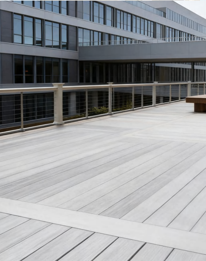
Skywalk Between Office Buildings
