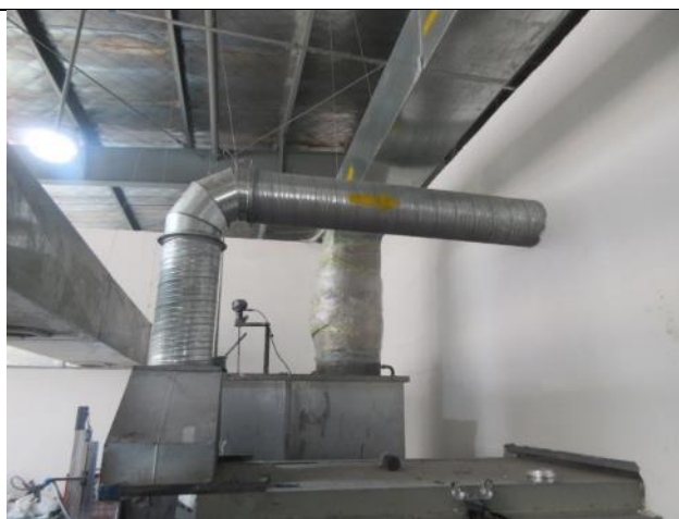
Collection Facility for Volatile Organic Compounds (VOCs) from the Spray Painting Process
