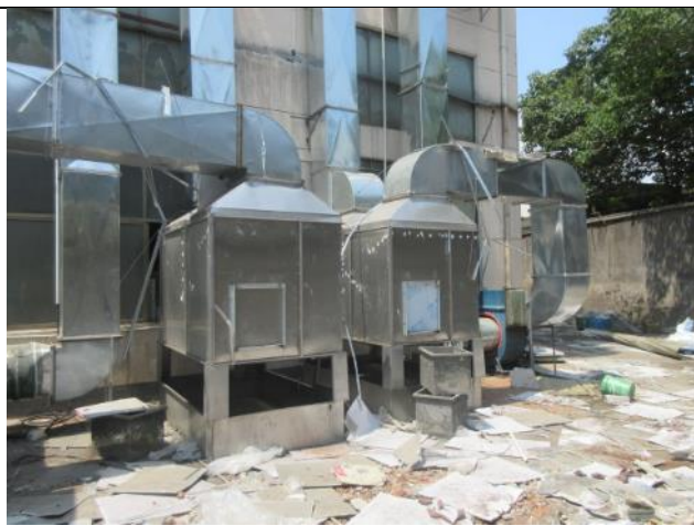
Wet Scrubbers for Dust from the Polishing Process
