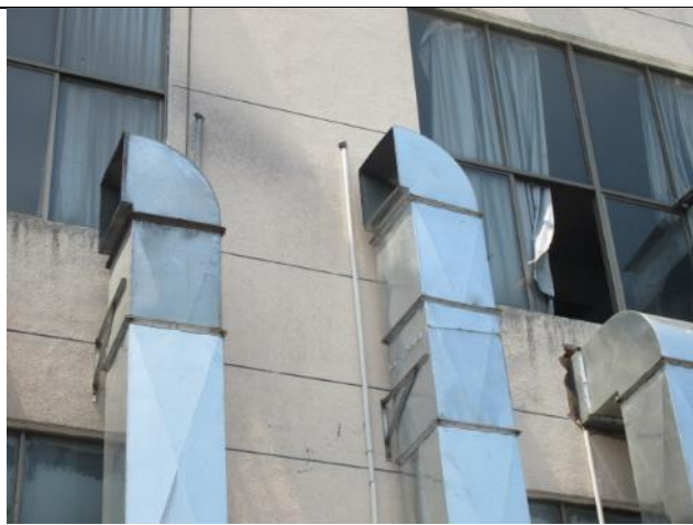
Discharge Outlets for Dust from the Polishing Process
