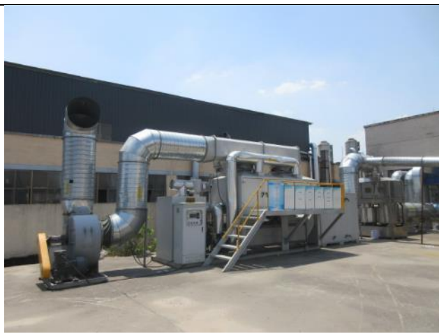
Wet Scrubber, Cotton Filter, Activated Carbon Absorber, Catalytic Combustion Facility and Discharge Outlet for VOCs from the Spray Painting and Screen Printing Processes, the Baking Channel of Powder Coating Process
