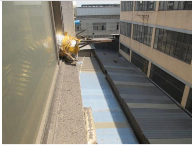
Discharge Outlet for Smoke from the Laser Marking Process
