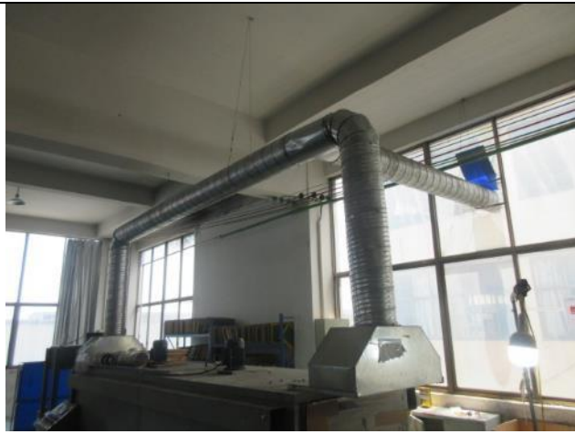
Collection Facility for VOCs from the Screen Printing Process
