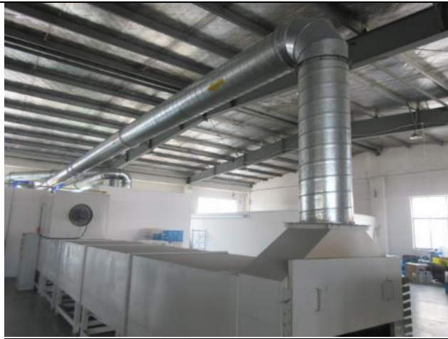
Collection Facility for VOCs from the Baking Channel of the Powder Coating Process
