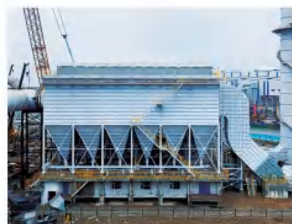
炼铁高炉出铁场除尘项目 Dust removal project of ironmaking blast furnace tapping yard
