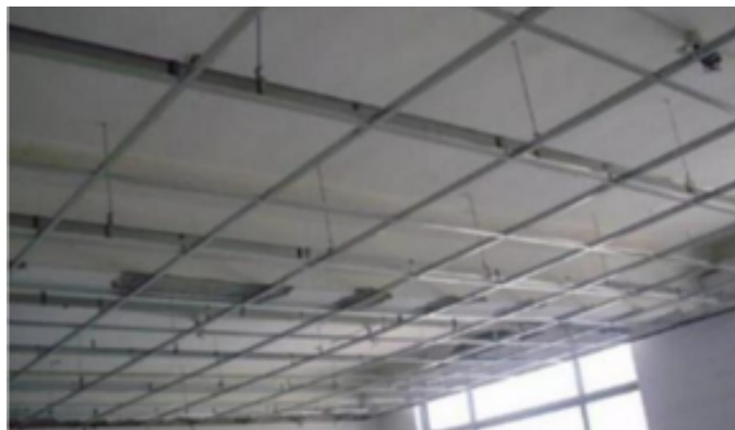
CEILING STEEL FRAME
