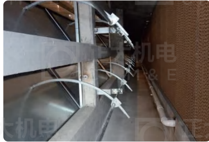
齿条开合进风门 Rack Opening and Closing Intake Door
