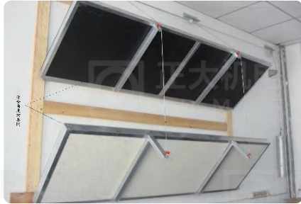
滑轮重力开合进风门 Pulley Gravity Opens and Closes the Intake Air Door
