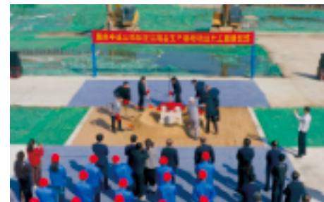
2024, Groundbreaking of the Aviation Daily Necessities Production Base.
