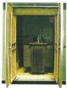
Transformer Compartment
