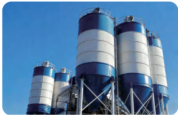
Concrete Mixing Plant
