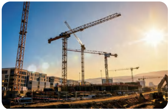
Construction Tower Crane
