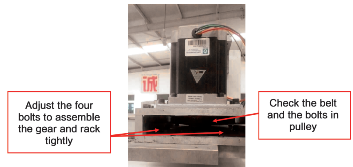
Fig.5 Checking the belt of X gearbox
