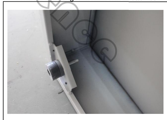
Photo of Leveling Bolt mounted in cabinet
