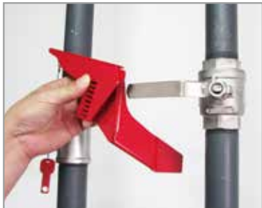
Step 1: Insert the ball valve handle
