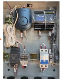
Pre-install & pre-wiring for PBAT-Gate, PBAT600Pro and HMI-Gate (optional)
